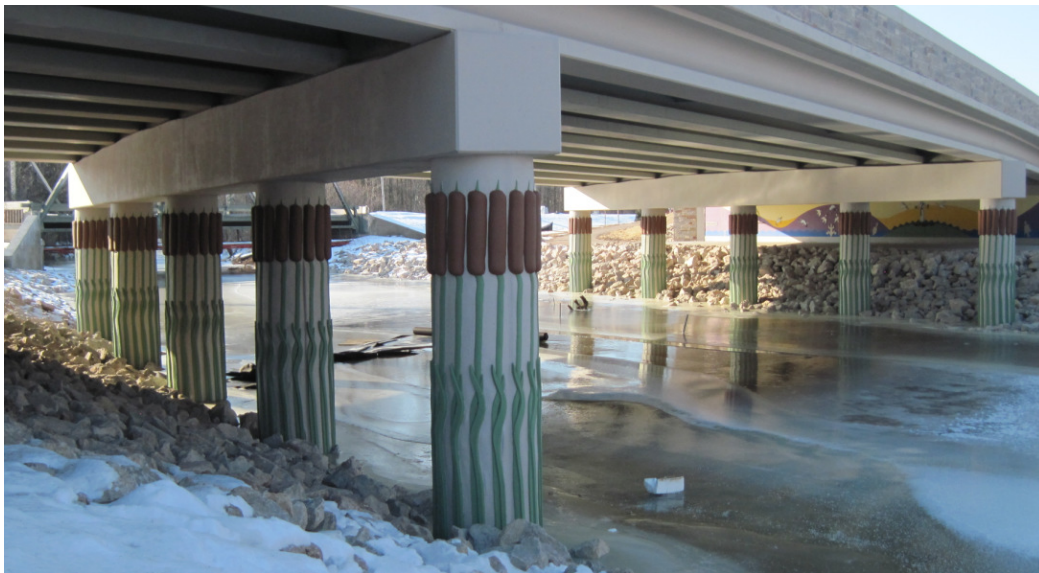
Figure 4 – Lightweight Elastomeric Medium Re-Use Custom Form Liners Create Graphic Bridge Piers (Wisconsin DOT - Oneida County)
