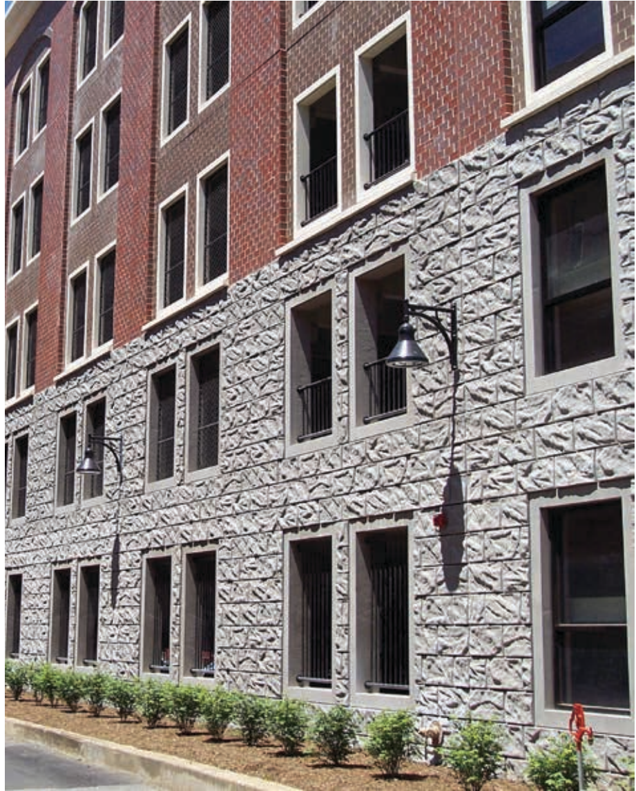
Figure 3 Chiseled limestone base for George Washington Auto Park, Winchester, Va.
